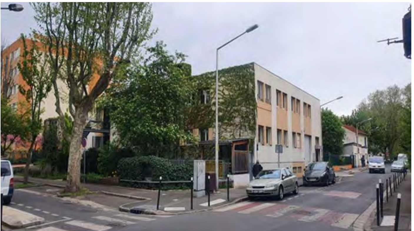
Picture of existing building (Halage)
