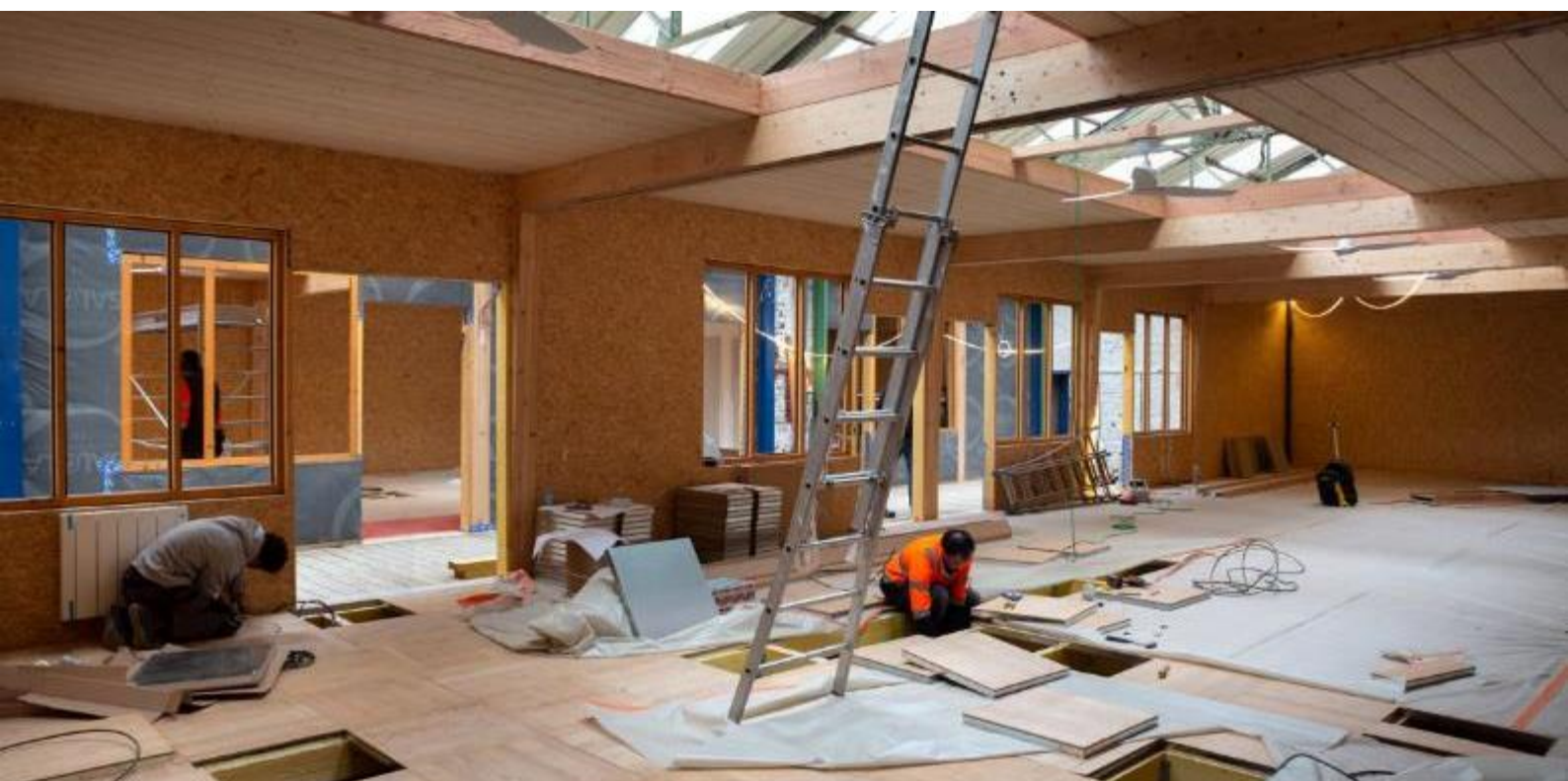
Renovation project, France, at l'Ile-Saint-Denis. Photo credits: Victoria Tanto
